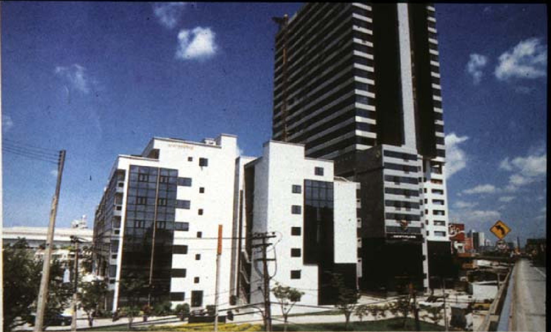
SSP Tower II & Mini Office at gateway to Port & Rama IV Road
